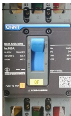
Figure 3.1-1 Lower electrical box plastic case circuit breaker (closed state)
