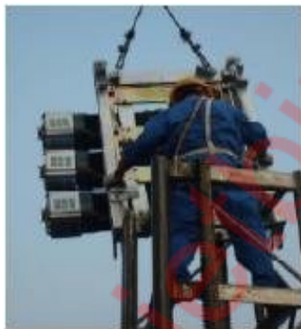
Figure 1.3-8 Erection of Drive System
